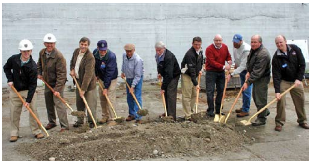
Puget Sound Rope groundbreaking of their new office space. Pictured are RH Construction owner and project manager, Mike Underwood (Underwood and Associates, architect for the project), Bill Short, Pat Mooney, Randy Longrich, John Dumas, Stuart Janke, and Dick Kilburn (Puget Sound Rope staff), Mayor Dean Maxwell and Brady Rowe, Port of Anacortes.
